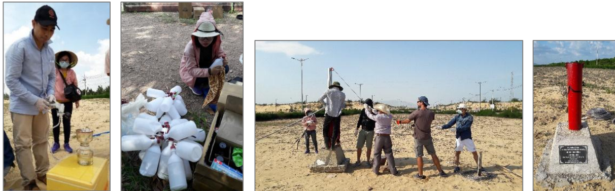
Filtering water samples on field (left); water sampling (centre left); installing pumping equipment in a monitoring well (centre right); groundwater monitoring well (right).
